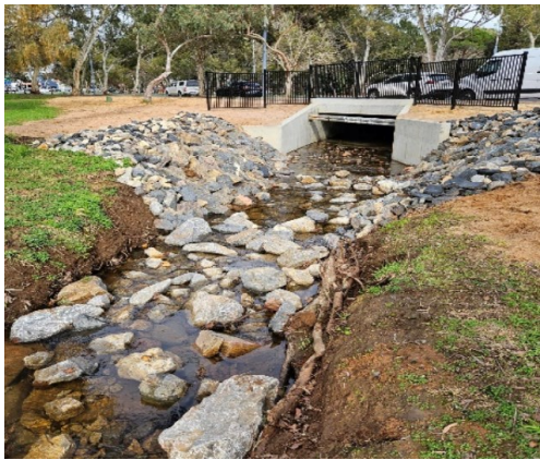
Unley Road Culvert Replacement
